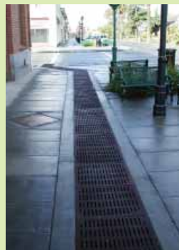
To decrease the potential cost of curb extension construction, trench drains can be used to allow pre-existing catch basin locations to be maintained. It is important to give proper proportions to trench drains. The smaller trench drain (center) is well proportioned and attractive, while the wide trench drain (right) is visually too dominant.
