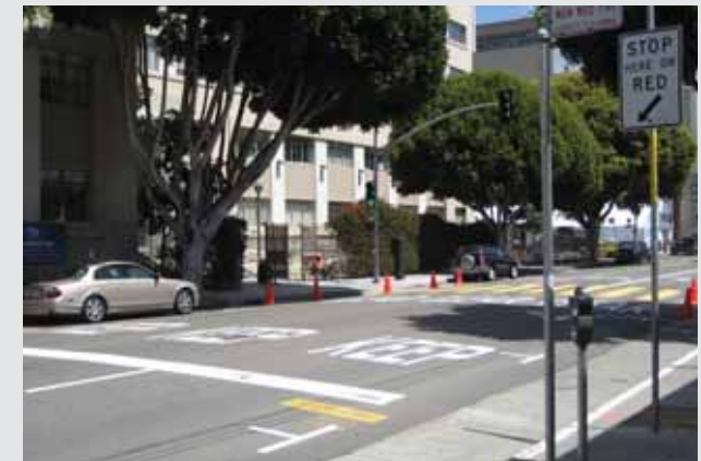
▲ Advance yield lines (top) alert drivers to an impending crosswalk; advance stop lines (bottom) require vehicles to stop in advance of a crossing
