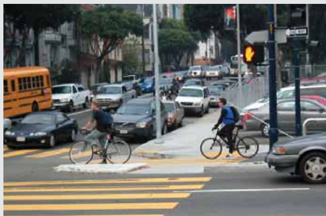
A center median island, right turn channel (corner) island, and side access lane median pedestrian refuge. (Source: Mike King)
