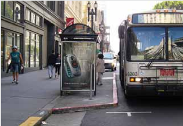
Curb extensions improve transit performance by allowing transit vehicles to load from the travel lane, removing the need to wait for a gap to re-enter traffic.
