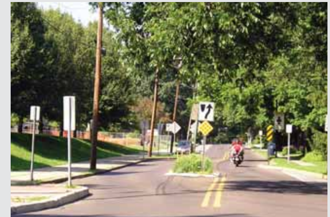
Chicanes slow vehicles by causing them to slightly change path. They add opportunities for landscaping to improve street aesthetics. (Source: Mike King)
