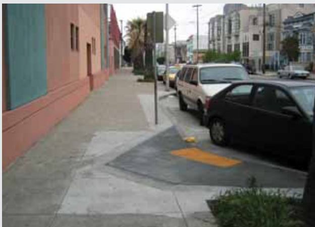
▼ A curb ramp should also be provided wherever on-street accessible parking is provided if it is not adjacent to a corner with an accessible curb ramp.
