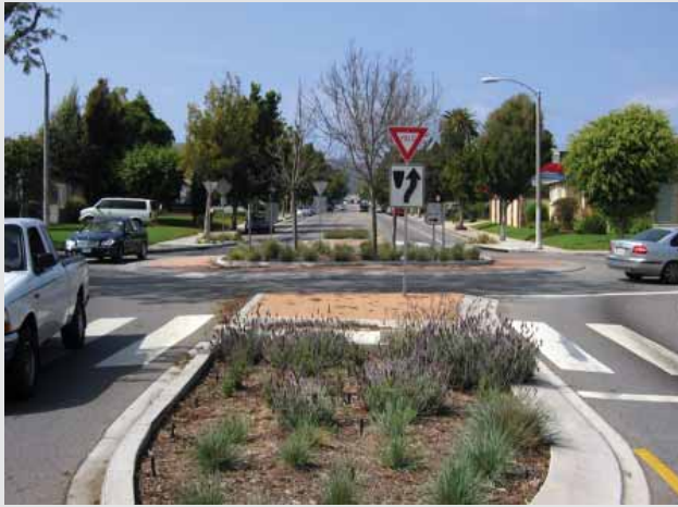
Roundabouts are typically larger and more formal yield-controlled intersections than traffic circles. The larger center island and multiple medians provide ample opportunity for planting and stormwater management.
