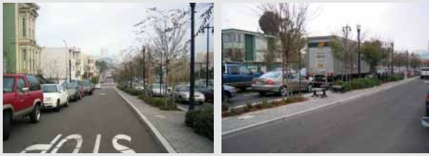
Side medians, such as those created on Octavia Boulevard, should be designed as pedestrian space. The local access lane should be designed similarly to reflect its orientation to pedestrians to provide a larger usable space for adjacent neighborhoods and businesses.
