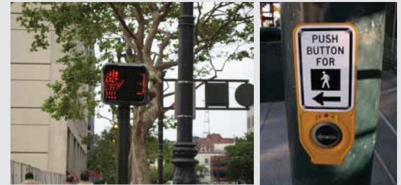
Pedestrian countdown signal and accessible pedestrian signal
