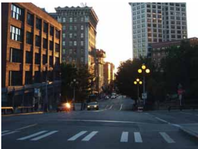
The staggered continental crosswalk increases crosswalk visibility but positions stripes to avoid vehicle wheels, reducing maintenance burdens
