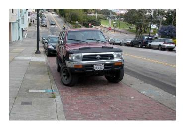
Attractive materials can distinguish the parking lane from other lanes. These pavers could be permeable, helping to reduce stormwater runoff.
