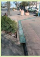
Trench drains may be used to allow pre-existing catch basin locations to be maintained and decrease the potential cost of curb extension construction. See Section 6.2 for appropriate use and design of trench drains.
