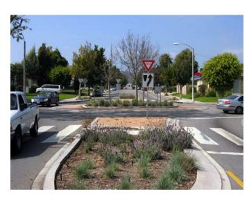
Roundabouts are typically larger, higher traffic volume intersections than traffic circles. The larger center island and multiple medians provide ample opportunity for planting and stormwater management.
