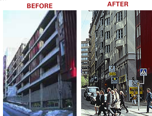
A new 'wall' with housing added to an existing parking structure. Stockholm, Sweden
