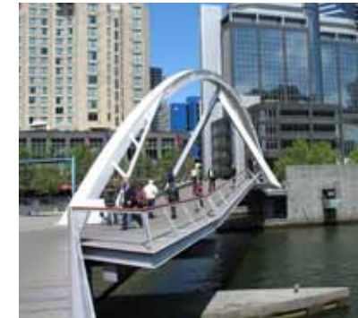
New footbridges connecting the piers form a complete water-walk. Bridges should be easy to open for the boats. Melbourne, Australia
