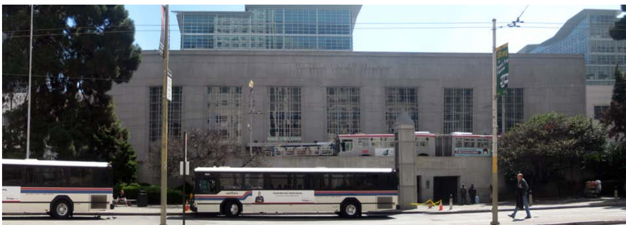
The existing Transbay Terminal is outdated and has a poor relationship to the street.
