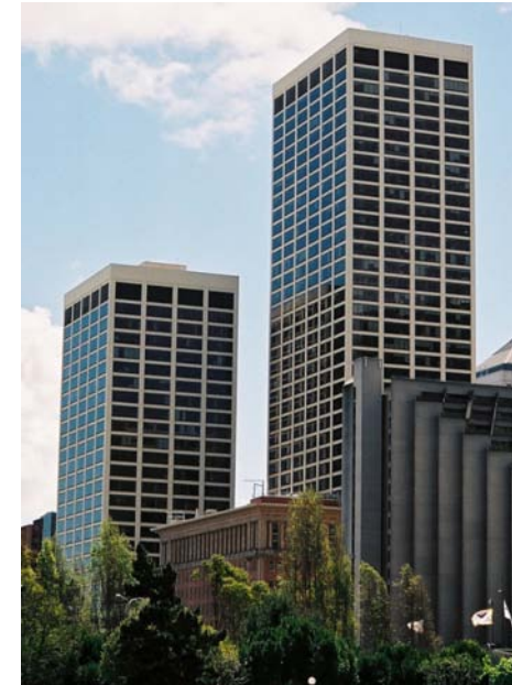
One Market Plaza has a 1.5 MW CHP system
