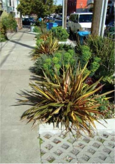
*Permeable pavement and stormwater-retention area incorporated into the sidewalk*
