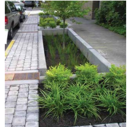
Portland bioswale on sidewalk
