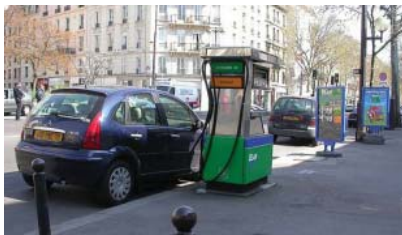
Single gas pump installed in sidewalk (France)
