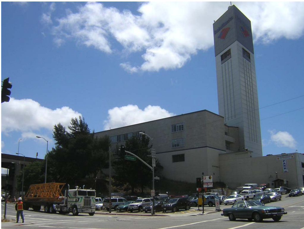
Viewpoint 2B - Bank of America Clock Tower, Harrison at First Street
