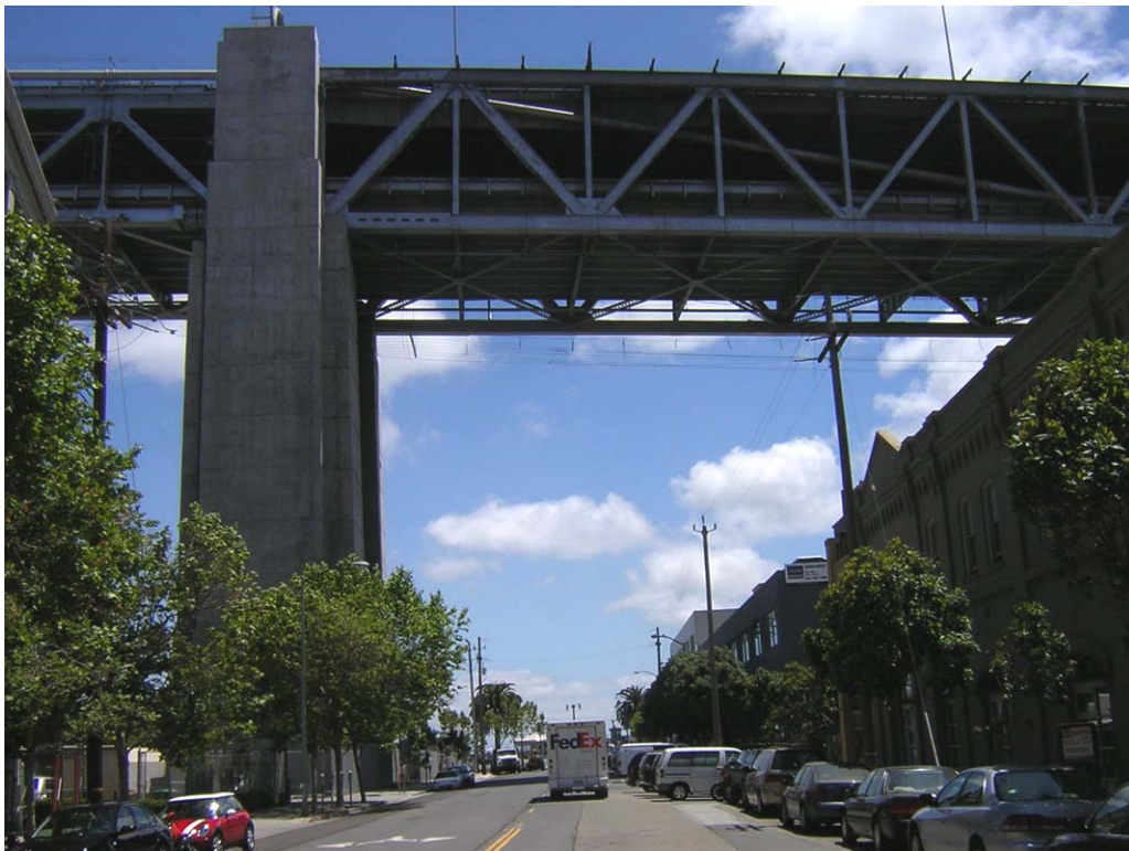
Bay Bridge anchorage and overhead span from Spear Street
