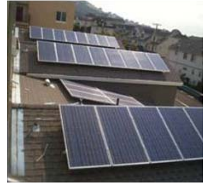
Solar panels can generate electrical energy on-site
