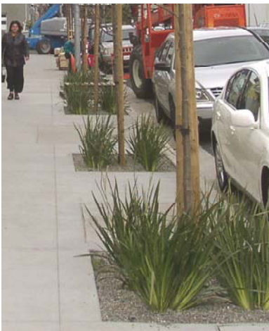
These natural tree wells are an example of how natural stormwater treatment can be incorporated into the street design
