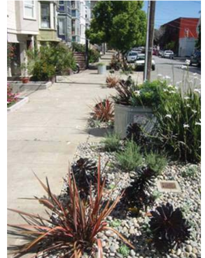
Permeable sidewalk features allow for stormwater to infiltrate
