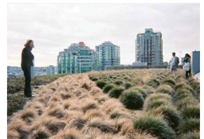
An example of a green roof
