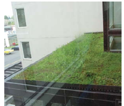
Green roofs have both environmental and aesthetic benefits.
