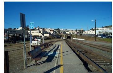
Existing Caltrain Station photo: EDAW
