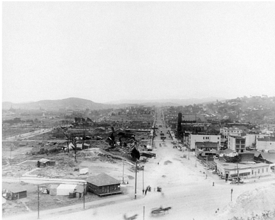
Figure 13. View of the destruction caused by the 1906 fire. This shot is looking down Dolores Street from Market. View south.
