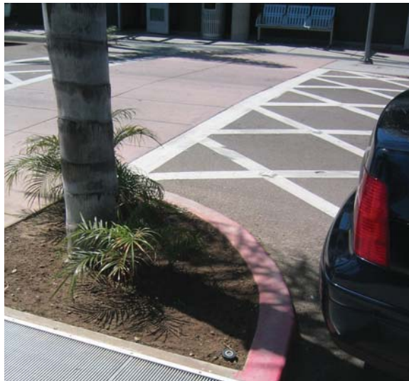
▲ Special crosswalk treatments may include a raised crosswalk, colored paving treatment, and trees in the parking lane
