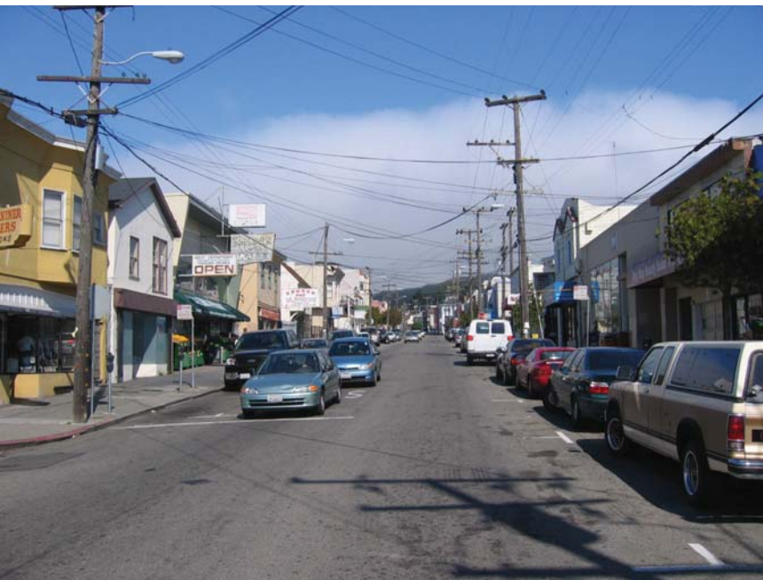
▲ Overhead utility wires detract from the aesthetic experience of the streetscape
