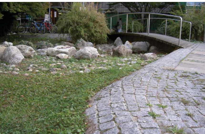
▲ Pathways across pocket parks and other large open space areas in the right-of-way can be raised to allow infiltration below Source: Sherwood Design Engineers
