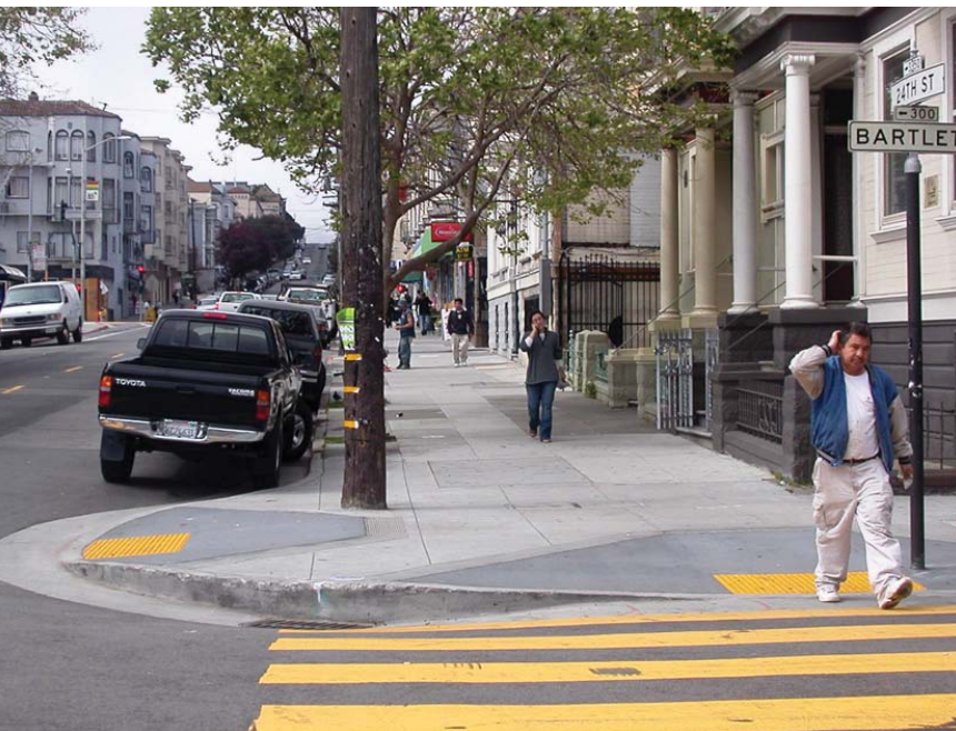
▲ Accessible curb ramps
