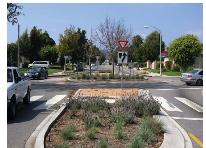
▲ Roundabouts are typically larger, higher traffic volume intersections than traffic circles. The larger center island and multiple medians provide ample opportunity for planting and stormwater management.
