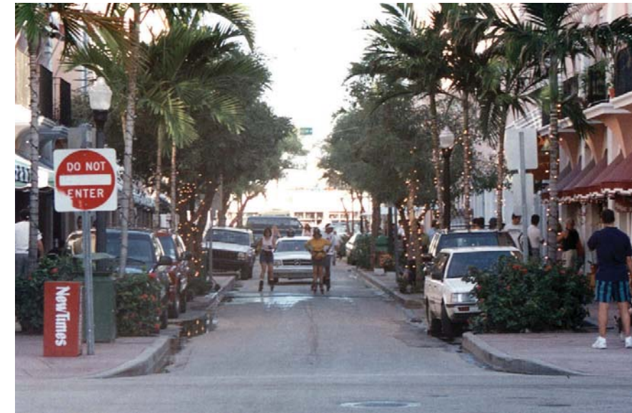
▲ Curb extensions shorten crossings and can act as a choker, narrowing traffic lanes at intersections to calm traffic, improving pedestrian safety at crossings
