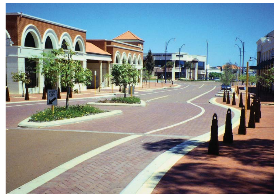
▲ Bollards protect pedestrians from passing traffic and can be an attractive streetscape accent
