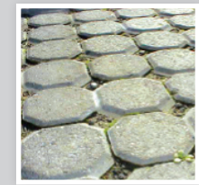
Special paving — entire right-of-way (6.4)
