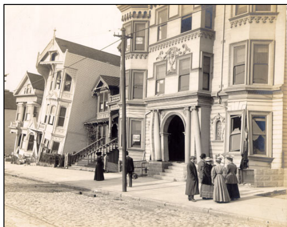
Earthquake damage on Howard Street between Seventeenth and Eighteenth Streets, 1906. Photograph source: San Francisco History Center, San Francisco Main Library.
