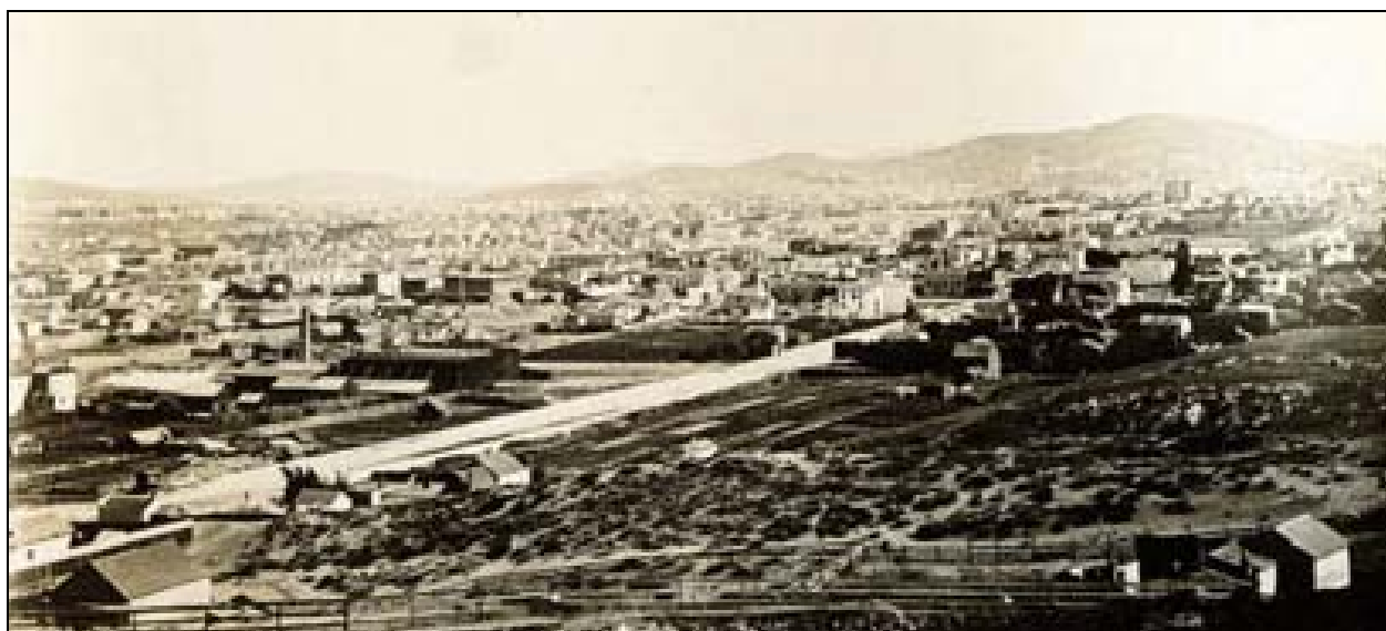
View southeast of the early suburban Mission District from upper Market Street, 1876. The street in the foreground running from Market appears to be Guerrero or Dolores. Photograph source: San Francisco History Center, San Francisco Main Library.
