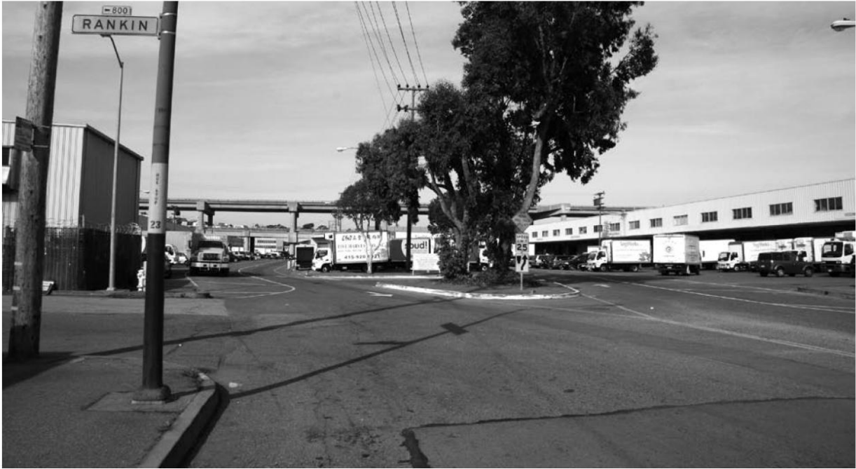
A. View Looking West from Jerrold Avenue and Rankin Street
