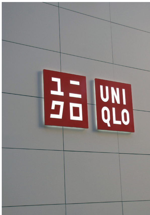
Example of an indirectly-lit sign with a shallow profile.
